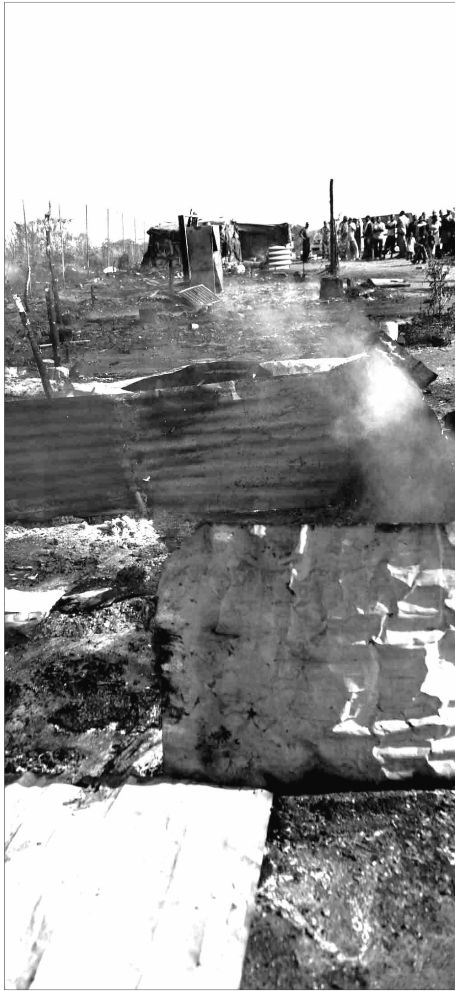
RISK: Masiphumelele needs a process called “re-blocking” to negotiate the removal of shacks to make space for firebreaks and storm water run offs, says the writer.
